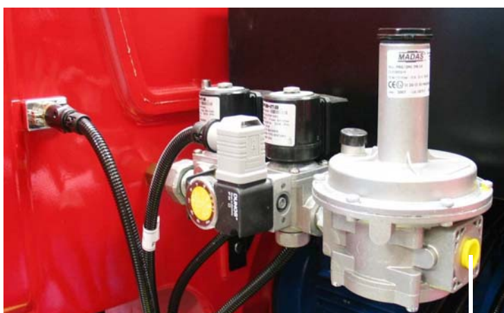
connection to the gas supply network 1/2"
