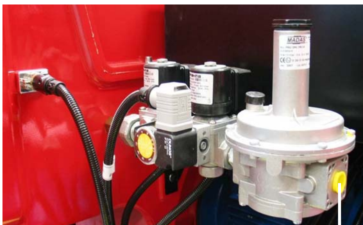
connection to the gas supply network 1/2"
