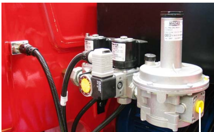
connection to the gas supply network
