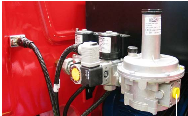
connection to the gas supply network - 1/2"
